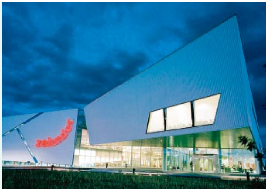
Zehnder Factory Zwolle for residential ventilation equipment
